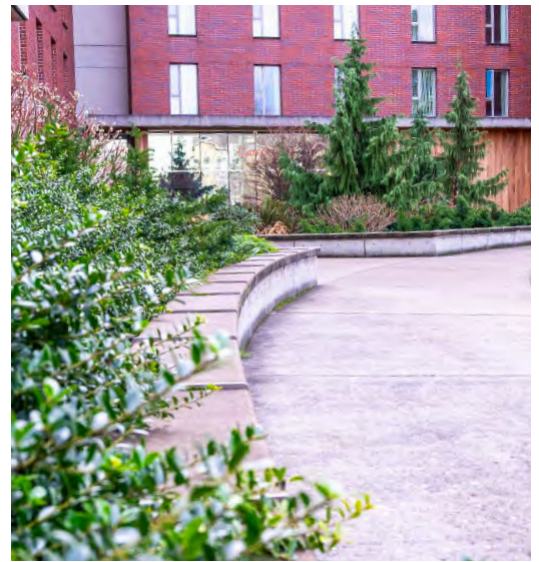
Rain garden on the northwest side of the International Living-Learning Center
