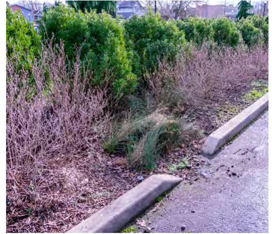
Bioswale on the northeast side of the International Living-Learning Center
