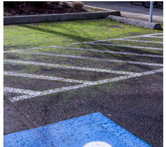
Permeable pavement on the northeast side of the International Living-Learning Center
