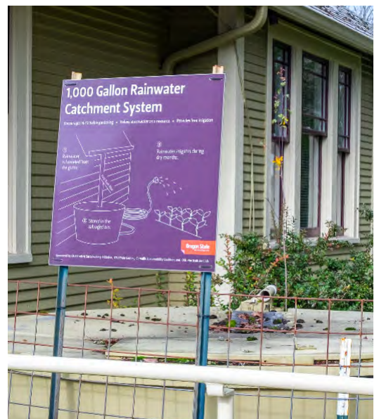
Rainwater collection tank on the southside of the Pride Center.
